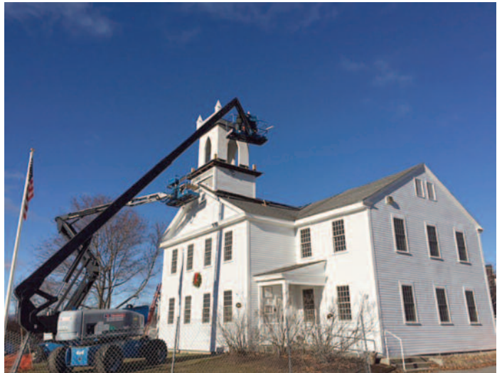
New London Town Offices under construction. Photo courtesy of Wendy Johnson.
