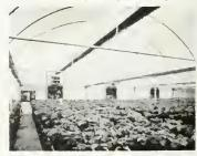
CO-RAY-VAC teatures burners in series beaming heat down entire tube length to plants and soil below.
