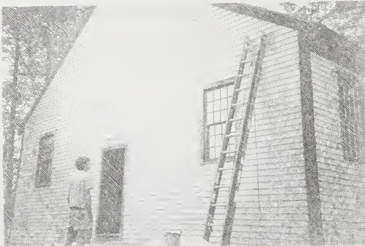
Eagle Scout Steve Kelley Working on 1772 Old Meetinghouse
