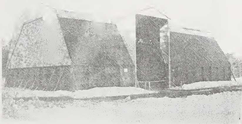
New Durham Highway Department Sand & Salt Building
