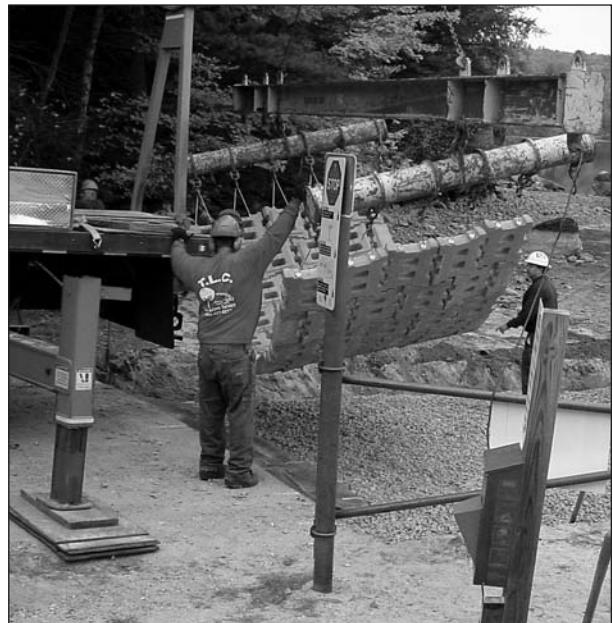
During the scheduled draw-down of Pleasant Lake, the boat launch was repaired using a mat made with fabric and stone, topped with blocks and then cabled together. By doing this work in-house, it saved the town about $35,000 and should help boaters get in and out of Pleasant Lake easier.
