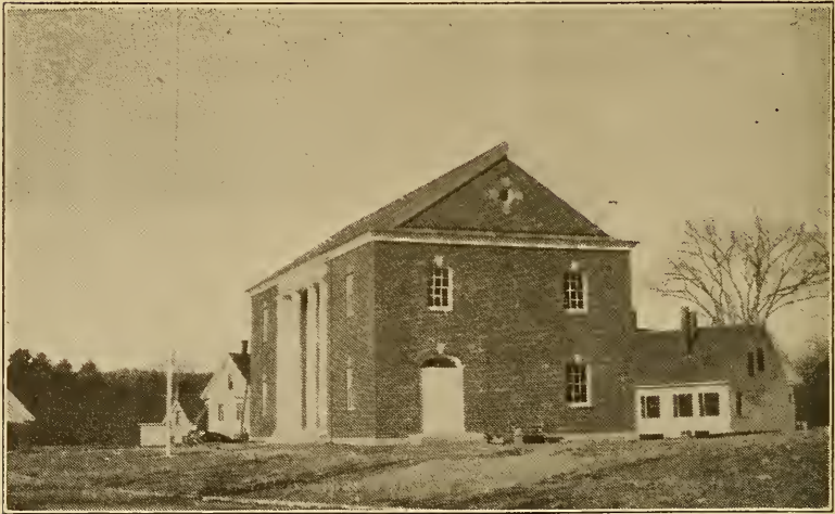
East End of the New Building
