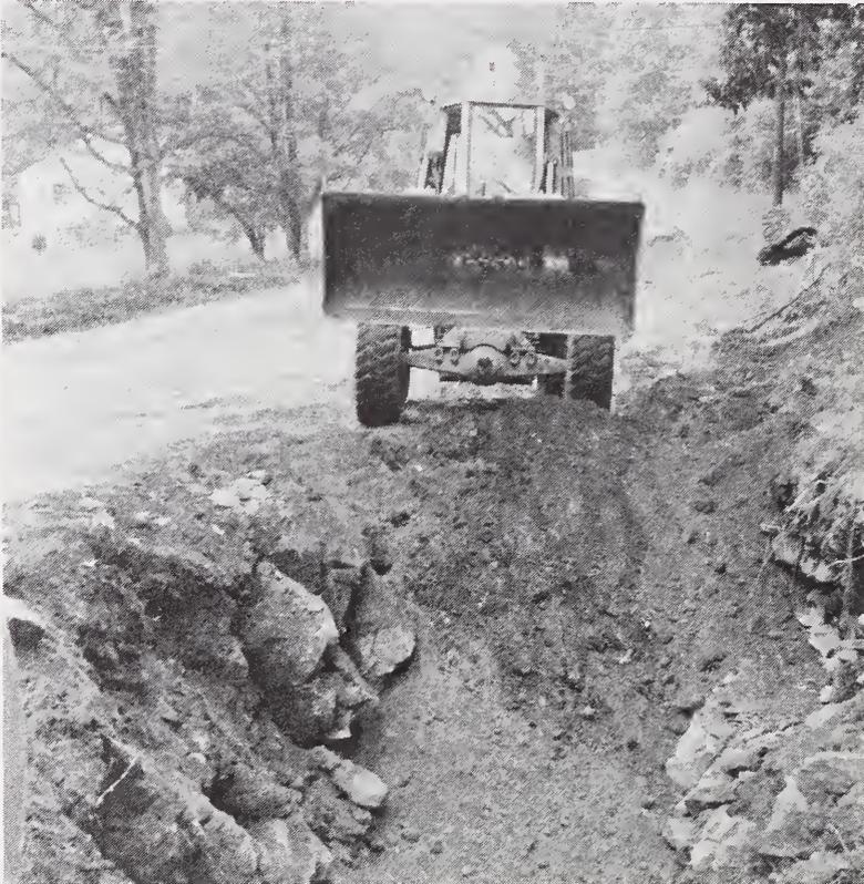
*WATER DISTRICT PROJECT – A front end loader from the United Construction Co. Fills in an excavation on Duncan Hill as part of the Meriden Village Water District's water main project. The new main and pumping system were constructed with grant and loan funds made available by the Farmers Home Administration.*
