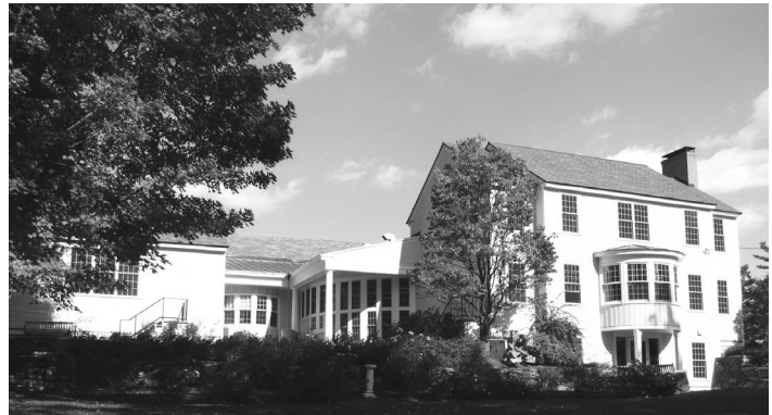
Newly renovated Tracy Library
