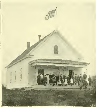
SCHOOL HOUSE DIST. NO. 1.
