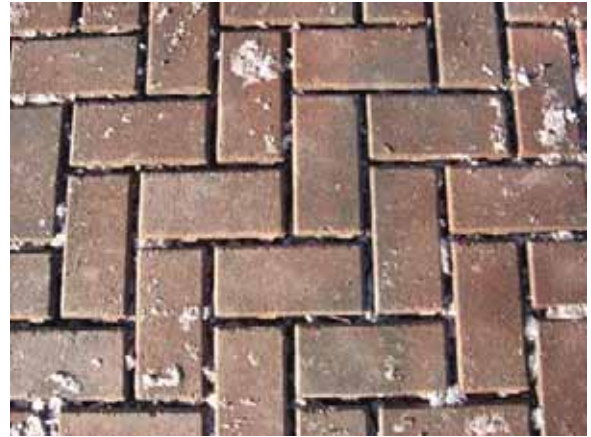
Figure 15: No. 8 joint stone has settled approximately 1 inch.
