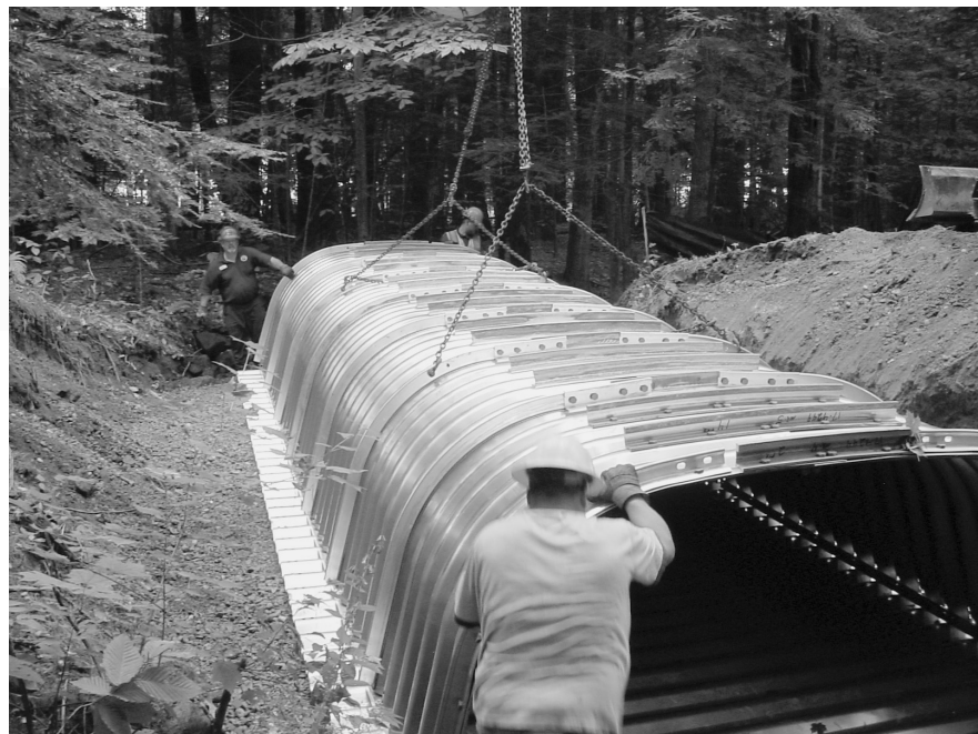
Mel Furbush (foreground), Mike Murphy (left), and Mike McElman guide the new culvert into place.
