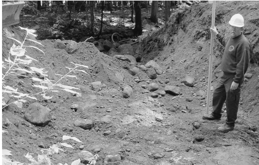
Foreman Bob Harrington sets the grade for the base of the new culvert on Lamson Lane.
