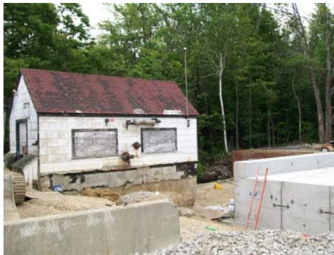
Pump House on Tricnit Road removed in 2009
