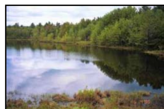
Flood Control Dam Dam Site 13
