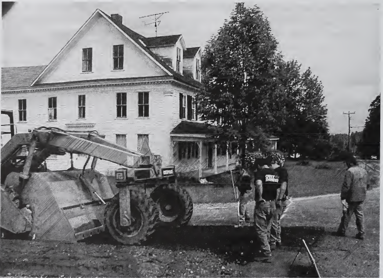
Allen Road Reclamation Project, 2000
