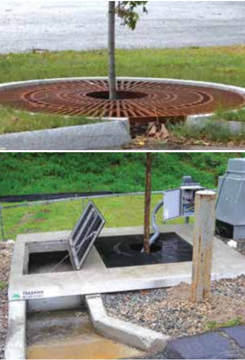
Though small, tree filters can manage runoff from the numerous lighter rain events that make up the majority of the annual rainfall in most regions. This makes them valuable assets in treating areas with large amounts of impervious cover.
