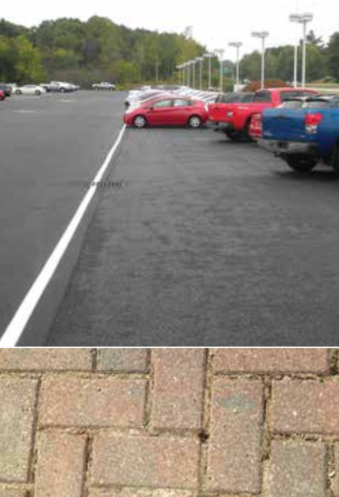
Permeable pavements like porous asphalt (above) and permeable interlocking concrete pavements (below) are powerful tools for addressing water quality targets in urban areas.
