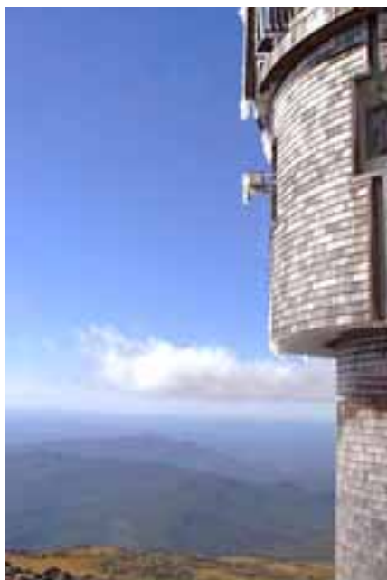
A springtime view of the Mt. Washington Observatory tower, in which all of the AIRMAP instrumentation is located. The project’s sample inlets are in the foreground. Photo by Kevan Carpenter
