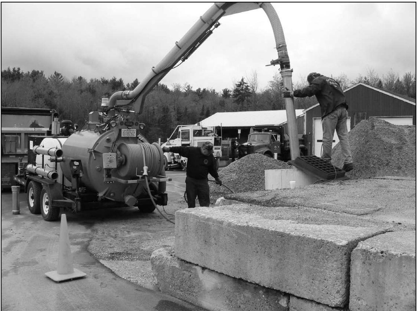
New London Highway Department members Mike Murphy (left) and Bob Harrington demonstrate the new catch basin cleaner at the Highway Department's May 2006 open house and building dedication.
