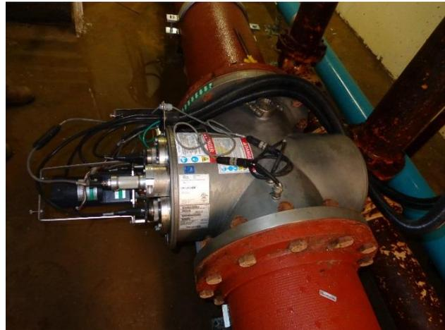
Figure 1a: This is a photo of the pilot UV disinfection system placed in Bethlehem. There are four UV lamps shown with black tops sticking out of the left side of the reactor. There are two UV wavelength sensors shown with longer gray columns connected to the black tops.
