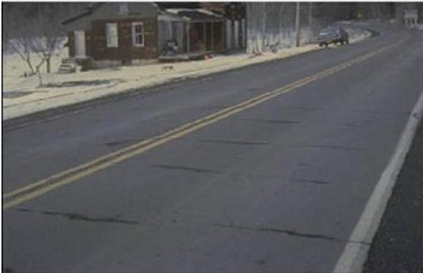
Here is an example of an asphalt pavement that has experienced thermal cracking. The cracks typically occur in a transverse direction and are spaced at regular intervals.
