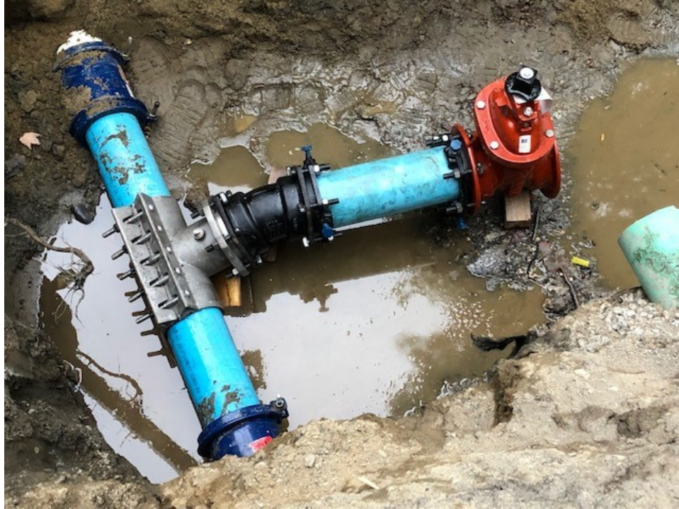
New service tap and gate valve for the ECA Maintenance Building.
