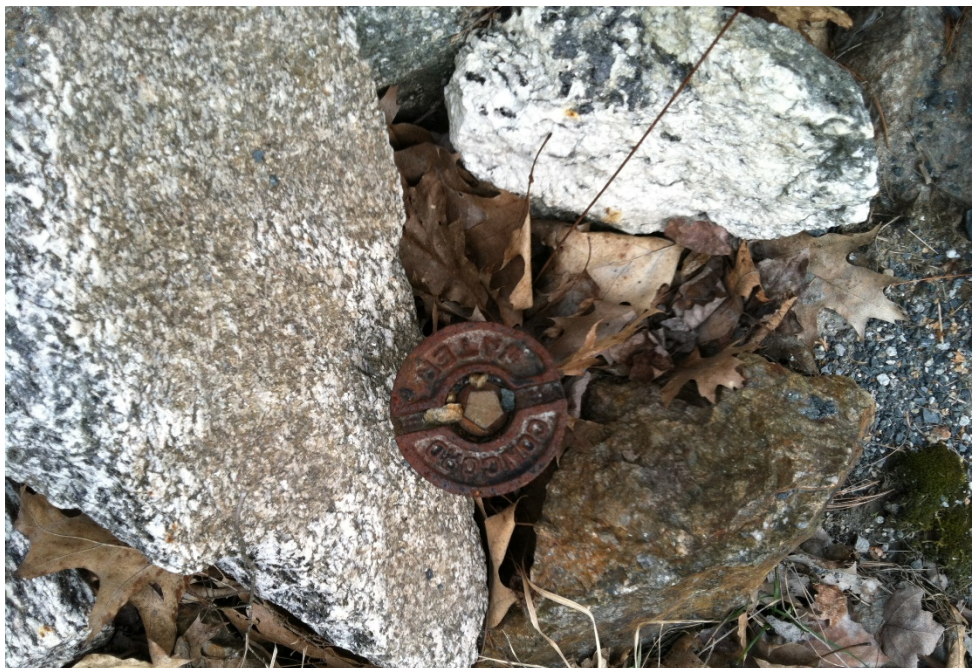
A minimum 5' radius (10' diameter) is required around all service curb stops. Rock walls like this will not be rebuilt should the curb stop need to be dug out for repair or emergency shut-off.
