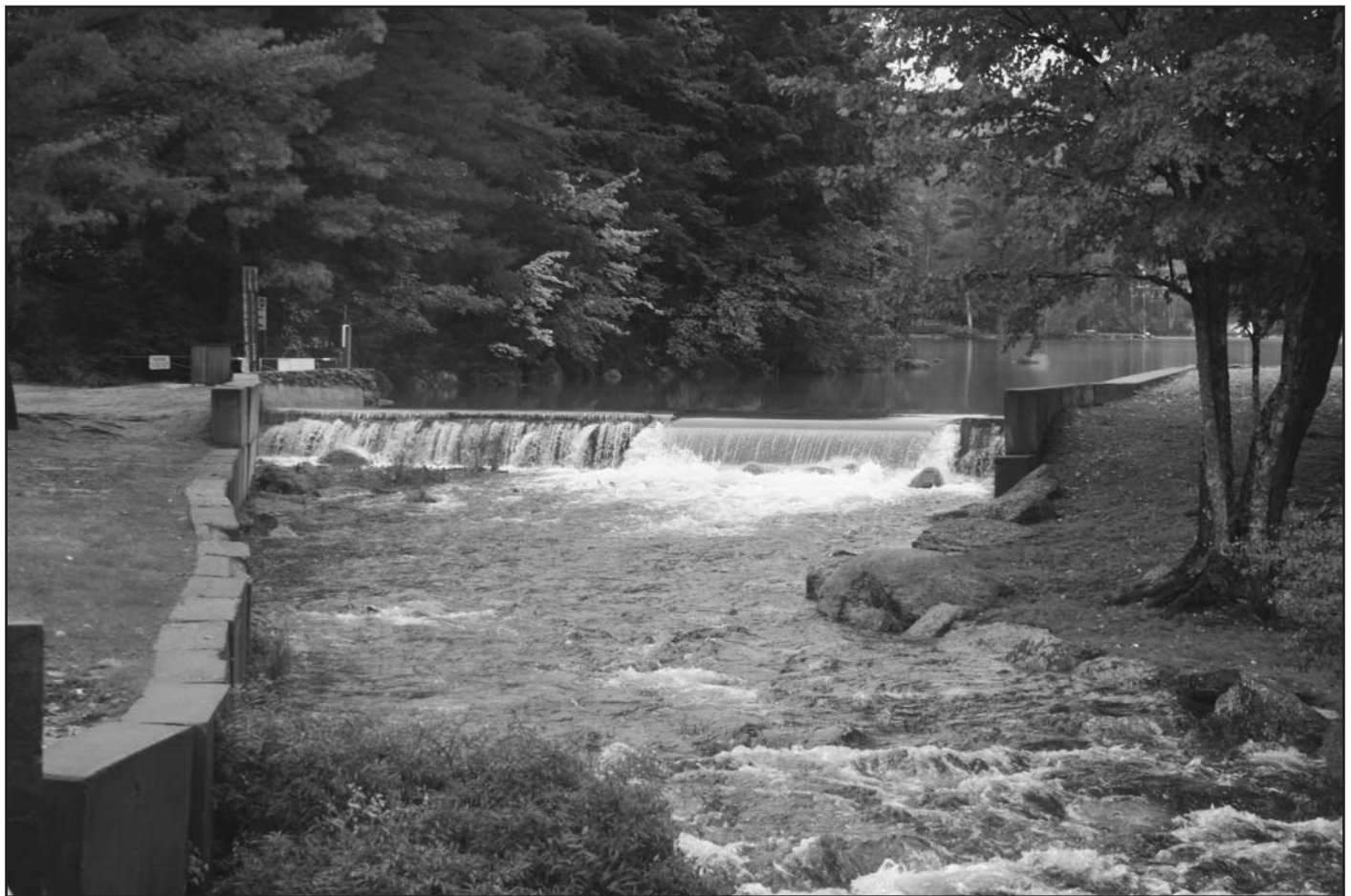
Spillway at Elkins Boat Launch, Pleasant Lake, October 2005.
