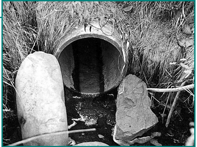
Overflow pipe on North Mill Pond
