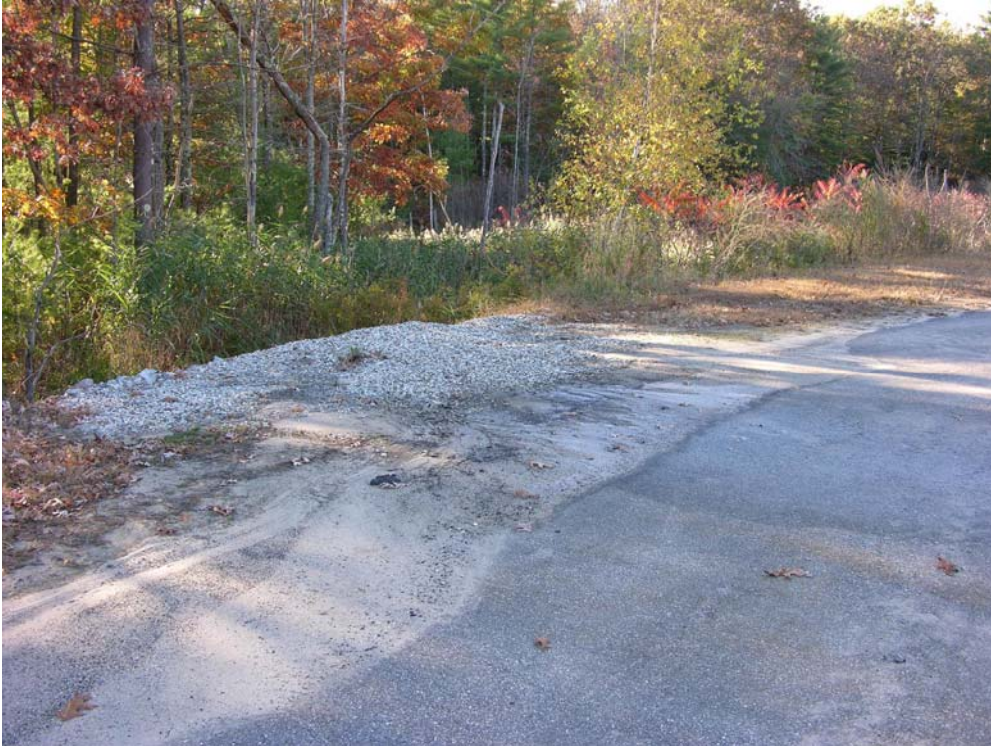
3. This photo shows where the water drains straight down into Wetland 31B.
