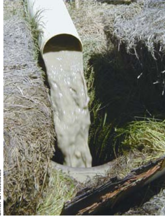
Drainage with heavy sediment load
