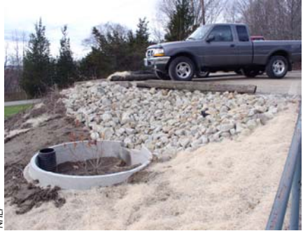
LID device treating stormwater from a parking lot
