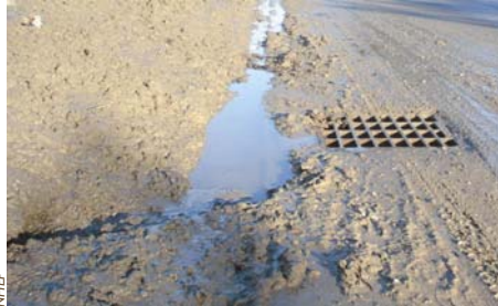
Construction site erosion near storm drain
