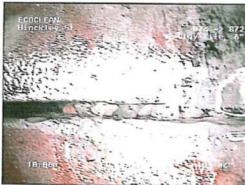
IMAGE: 12b, TAPE #: 11/29/2005 102.9FT, offset joint, slight
