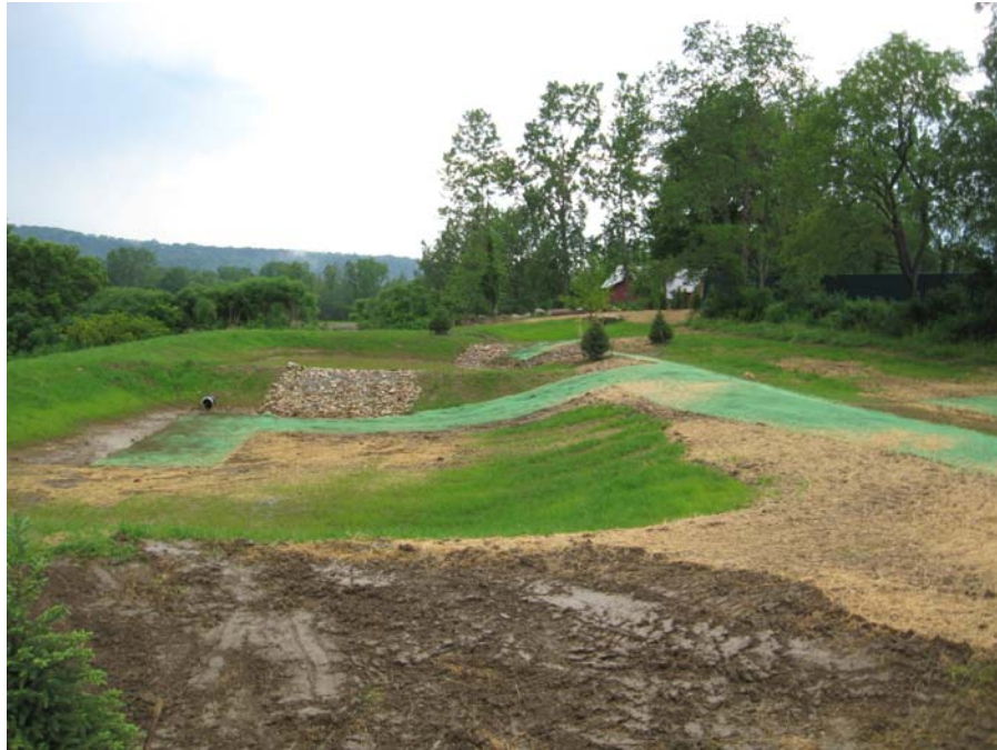
Surface Sand Filter Under Construction. Note Detention Pond in Background.
