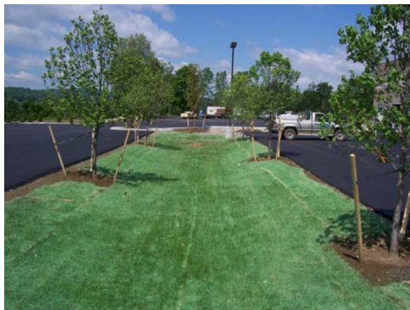
Bioretention Area Within a Parking Lot.
