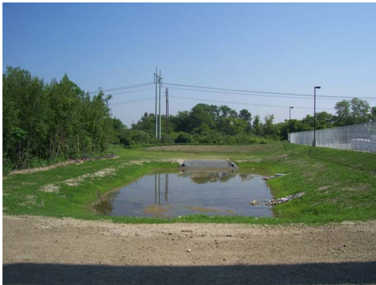
Small Detention Pond at an Industrial Facility
