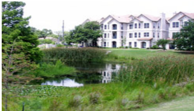
Photograph showing stormwater Pond City of Austin, Texas.
