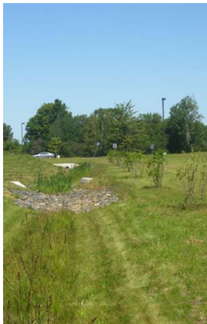
Buffer and Grass Treatment Swale.
