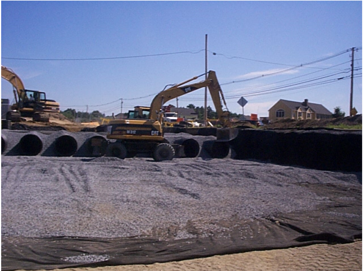
Large subsurface infiltration system under construction.
