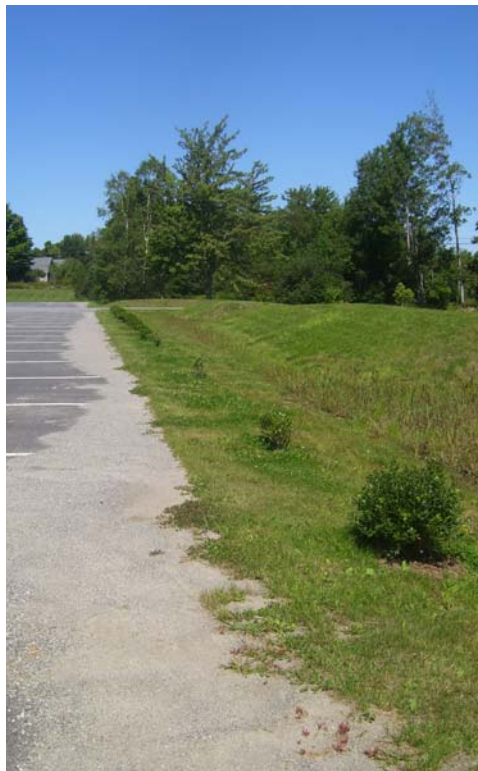
Grass Treatment Swale at Edge of Parking Area.
