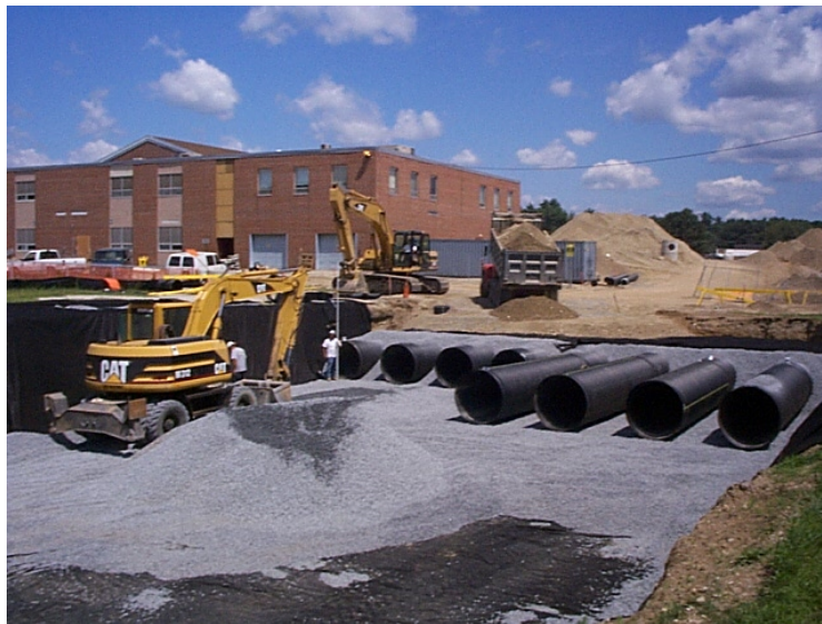
Photograph of large infiltration practice which serves as both quantity and quality practice.
