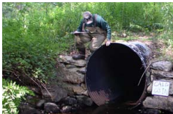
Researchers assessed 110 culverts to provide data for a computer model that will help municipalities update infrastructure to accommodate changing climate conditions.
