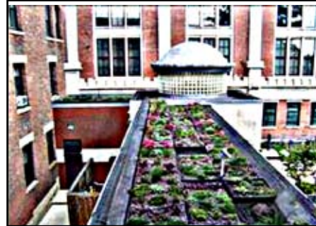
A greenroof installed on City Hall in Manchester in 2002.
