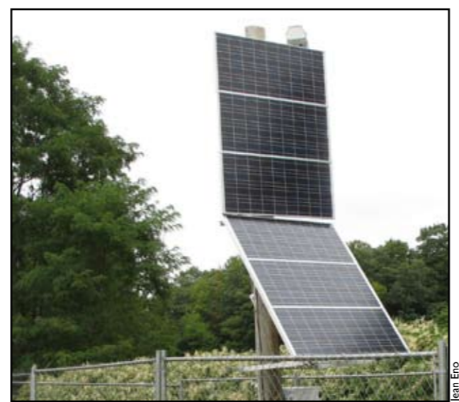
Large solar panels erected near Rt. 33 power a video camera aimed at the Winnicut Dam that can be viewed online at www.earthcam.com/winnicut to watch the dam removal process.
