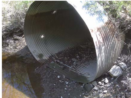
Downstream (bayside) outlet
