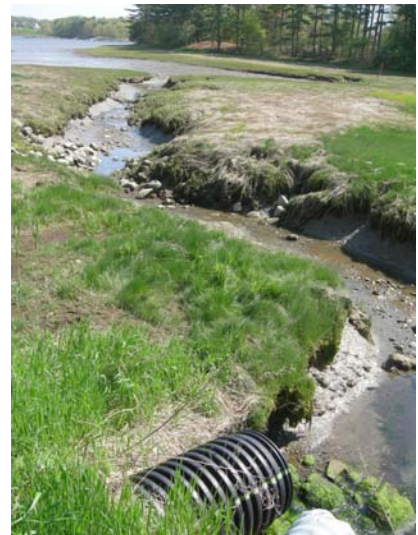
Stormwater outfall to Spruce Creek
