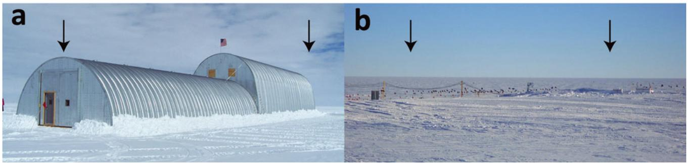
**Fig. 2.** (a) View of the core-handling (left) and drilling (right) arches in January 2006 shortly after construction. Both arches are now completely buried by accumulation and drift. (b) The core-handling (left) and drilling (right) arches at the end of the 2012/13 field season, after seven winters of accumulation and drift. The arrows in each photo point to the ends of the arches.
