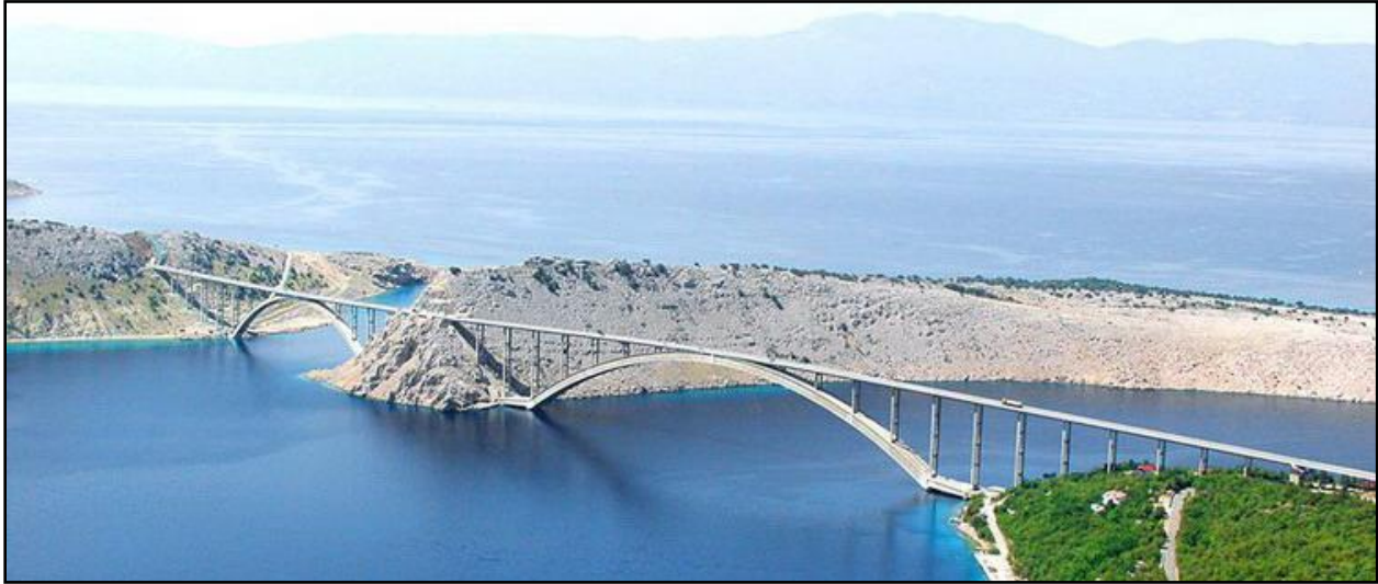
Figure 29: Krk Island Bridges
