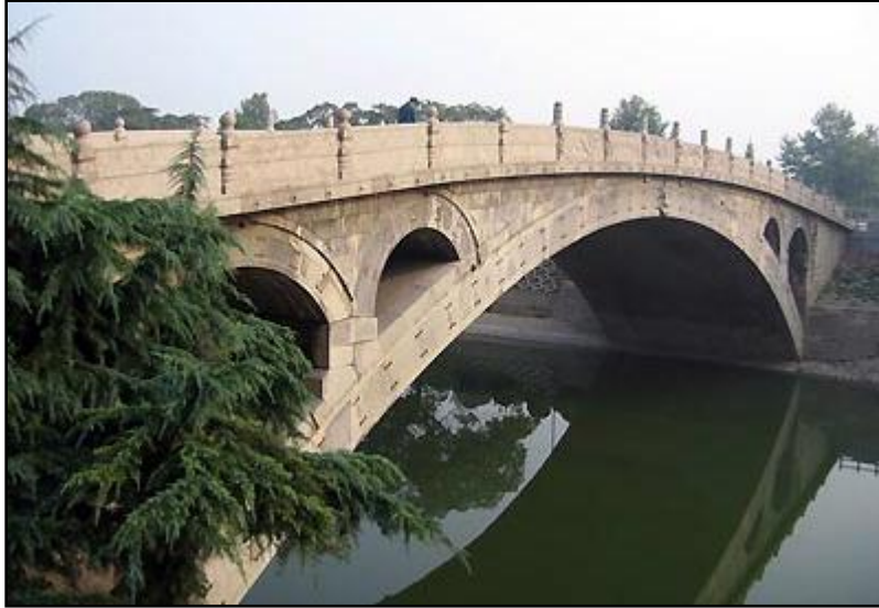
Figure 18: Zhaozhuo Bridge ( http://www.topchinatravel.com/china-attractions )
