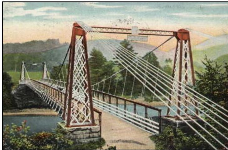
Figure 64: Suspension bridge in West Chesterfield
