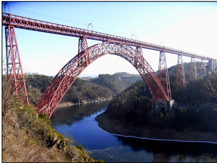
Figure 20: Garabit Viaduct ( http://www.flickr.com/photos/daviddb/2140318177/ )
