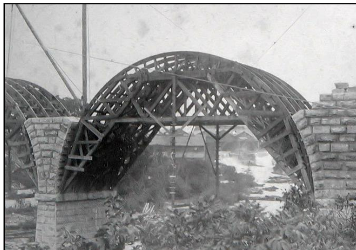
Figure 40: Wood centering for a masonry bridge in Minneapolis
