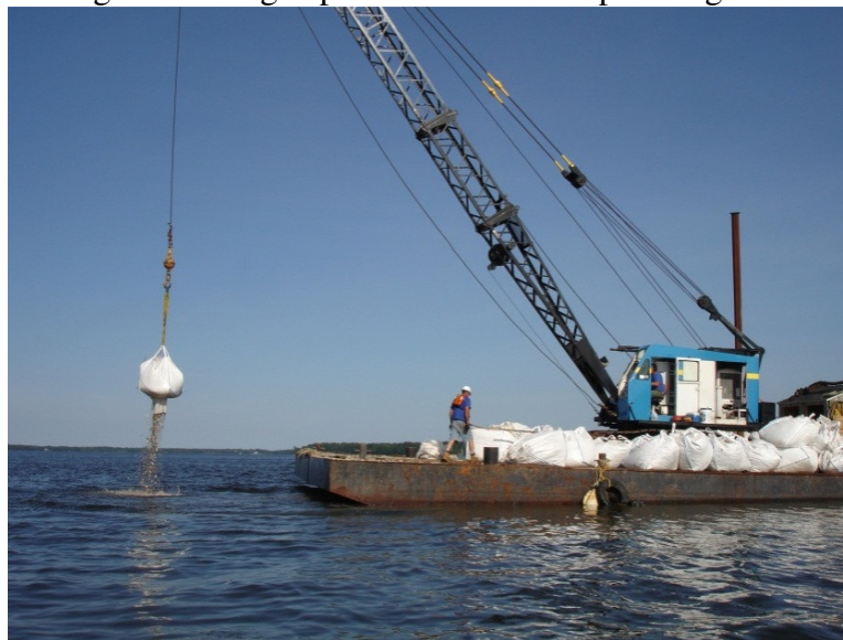
Figure 8. Barge operator with crane spreading shell
